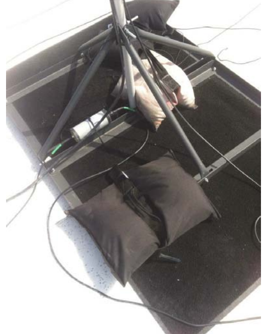
Non Penetrating Roof Top Mount with sandbags. Radiowavz RF Choke
