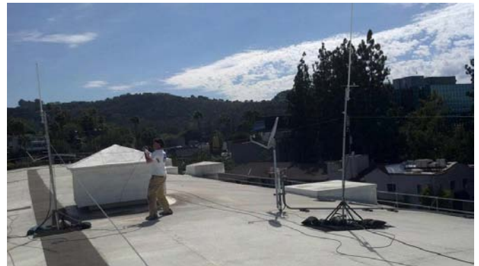
Installing the antennas
