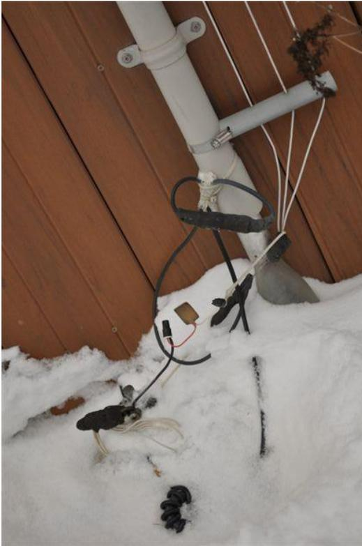
Base of Antenna. Feed line is black and attached to the base of the tower along with vertical stub wires at the wine bottle. Coax shield is attached to the capacitor with Marettes and then to the ground rod and radials. The feed line is wound around the toroid partially buried in the snow at bottom of photo, before going on to the base of the antenna at the wine bottle.
