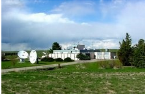
The WWV complex in Fort Collins, Colorado. [NIST photo]
