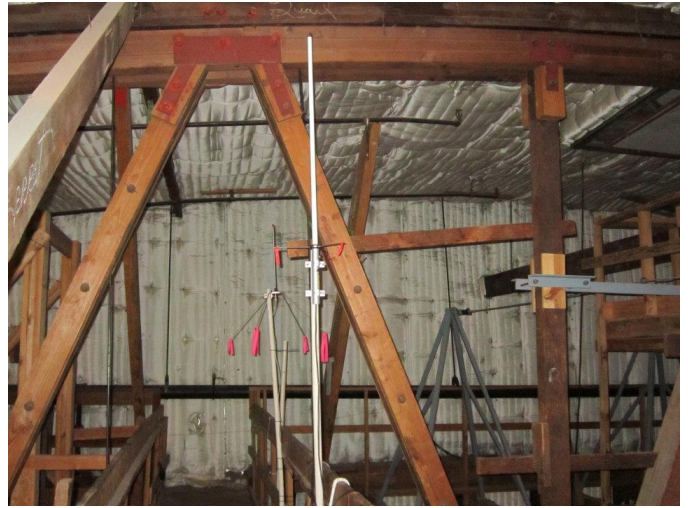
Arrow Antennas GP146 and GP435 also mounted in the rafters of the sound stage.
