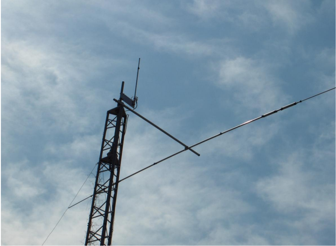
I noticed the other 2 sets of elements available on site.
