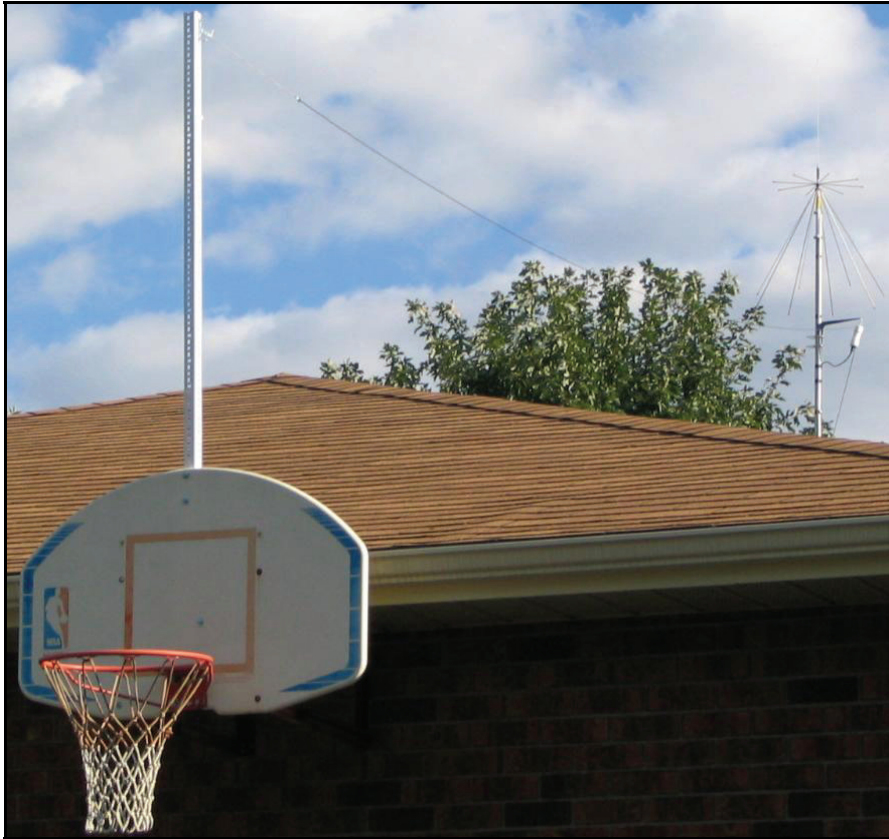
Front of house with 6ft T-bar riser for Windom
